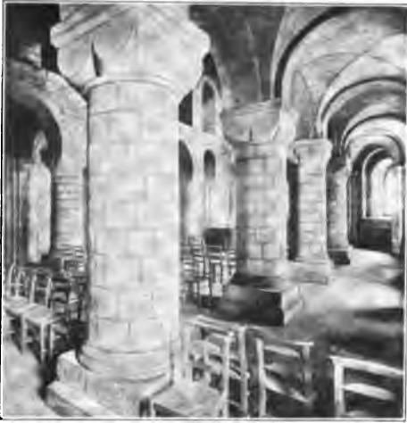
Fig. 13. —Intersecting Groined Vaulting. Early Example. St. John's Chapel, Tower of London.
