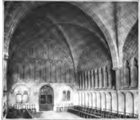
Fig. 14. —Intersecting Ribbed Vaulting. Late Example. Chapter House, Bristol Cathedral.
